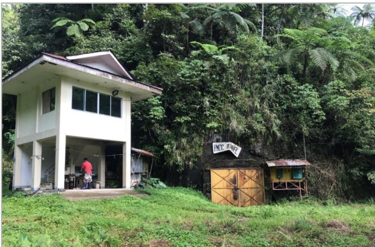
FIGURE 1: PMDC Victory Tunnel Project adit (Diwalwal Gold Project).
